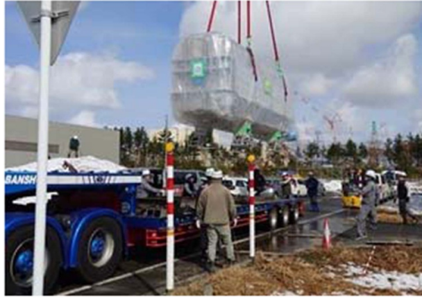
Figure 10. Loading of the cryomodule on the articulated lorry. Reproduced from [20]. CC BY 4.0.
