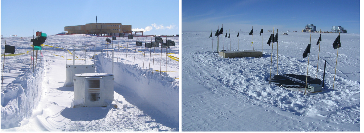
Figure 4.7.: Images of one IceTop station during (left) and right after deployment (right).
