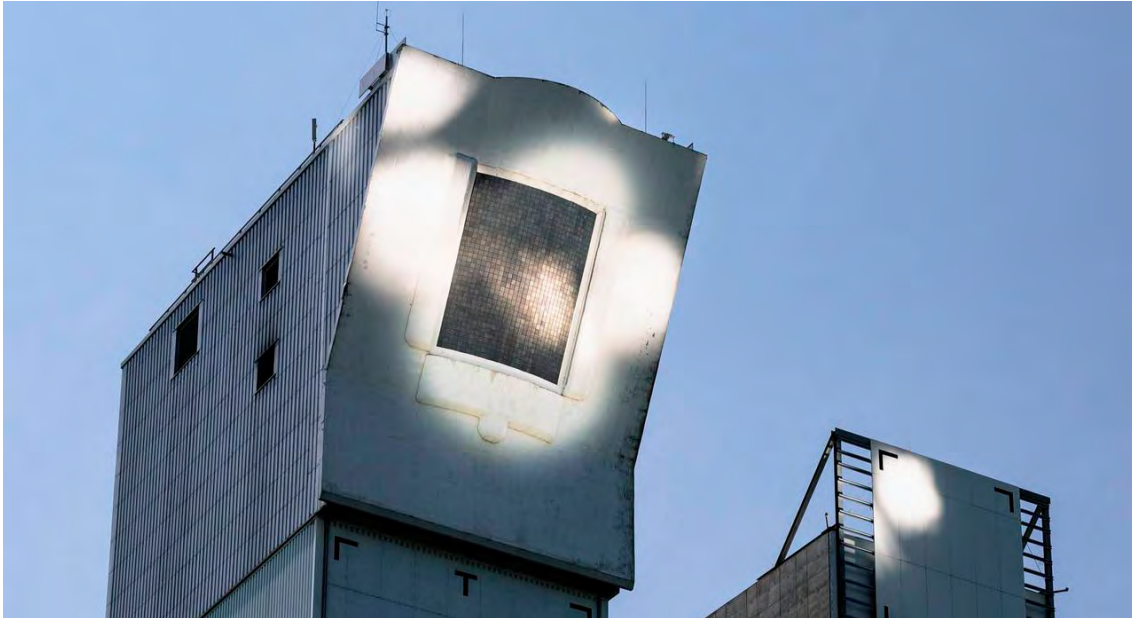
Figure 2: The two concentrating solar power plant towers in Jülich. They have been operated since 2009 and 2011 respectively. Till today, there is active research to avoid energy spillage (left) and miscalibration (right) using modern data-driven methods.
