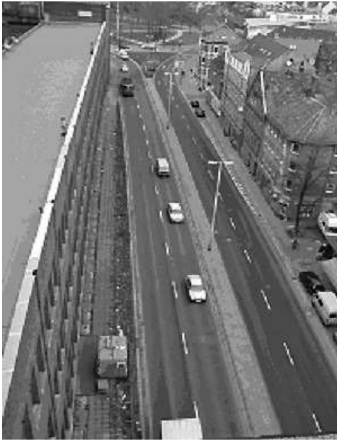
Figure 1: Göttinger Strasse in Hanover with location of three in situ measurement systems inside the street canyon (container). The roof-top station is near the position of the photographer.
