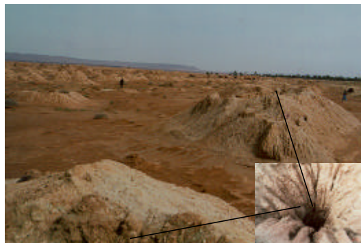
Fig. 3 : Craters, each marking the mouth of a qanat shaft in Southern Morocco. Groundwater from the Higher Atlas mountains is directed to an oasis in the plains (Photo Prinz)
