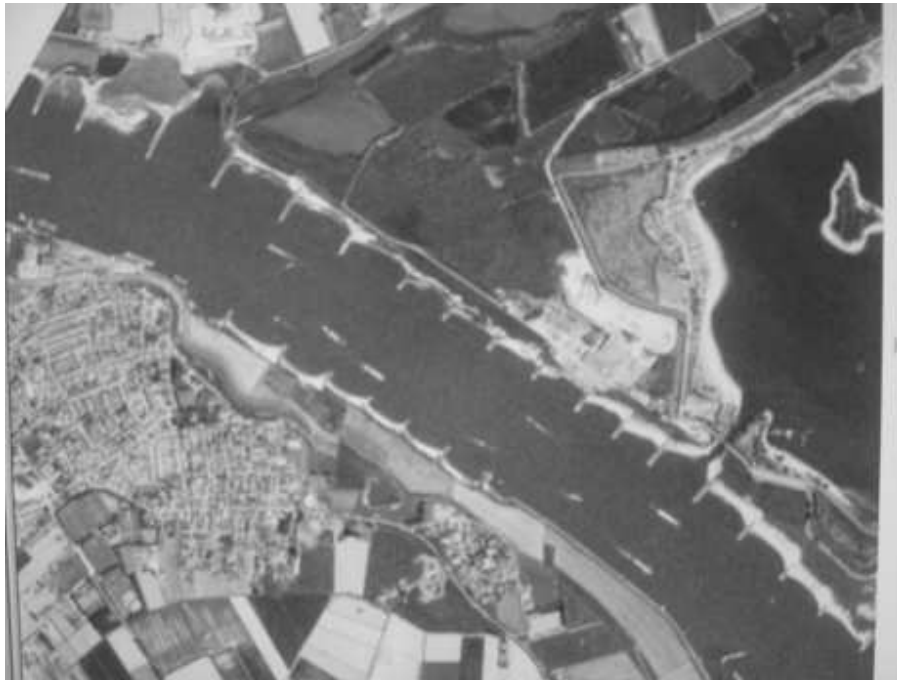
Figure 2.4. Aerial photograph of groin fields in the River Rhine close to Emmerich showing the density of the shipping traffic
