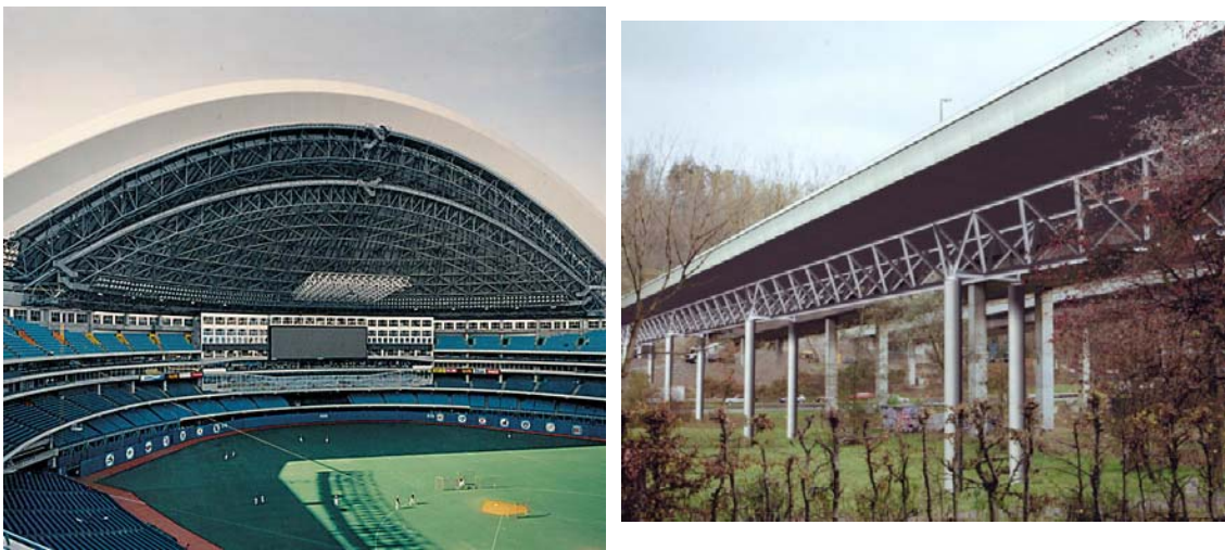
Figure 2 Toronto SkyDome roof structure and the Baregg bridge in Switzerland
