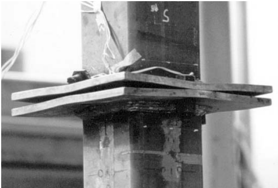
Figure 2.13 Square flange-plate connection (S4-1) with four bolts after failure
