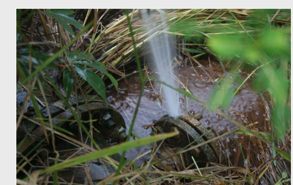
Dilapidated pipeline
