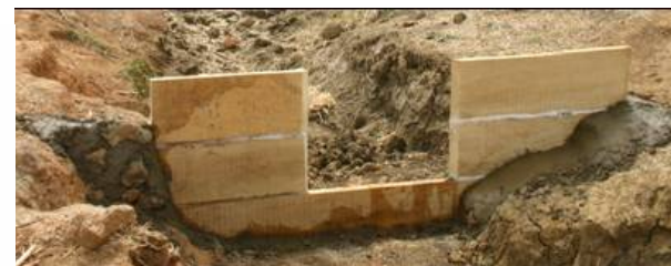
Installation of small weirs Q = f(h)
