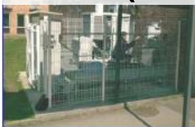
A PlugPower natural gas fuelled CHP unit powers a greenhouse in Nancy, France.
