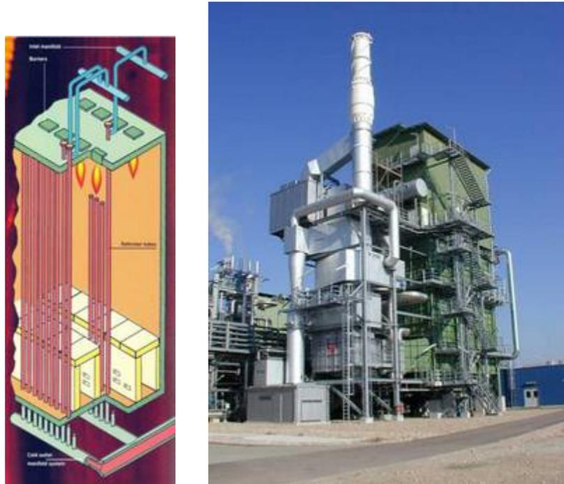
Figure 9: Cut through the primary large scale reformer and a view on a Linde-Natural Gas-Steam-Reformer (H<sub>2</sub> capacity 35.000 Nm<sup>3</sup>/h, purity after PSA 99.99 %)
