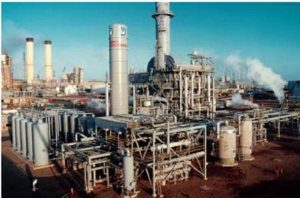
Figure 11: Large scale industrial SMR with PSA and storage
