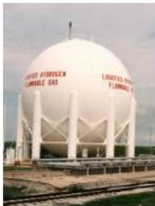
Figure 35: 3800 m3 LH2 Storage at Kennedy Space Flight Center in Florida (Source NASA)
