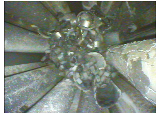
1100 mm: debris relocated downwards from removed nine test rods
