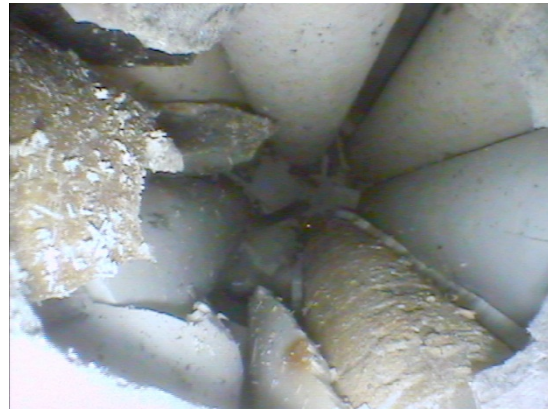
view through the empty cladding
