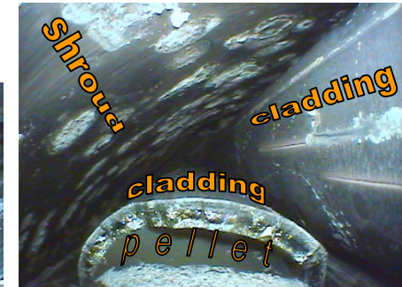
900 mm: circumferential and longitudinal cracks at the cladding; nodular breakaway corrosion at the shroud
