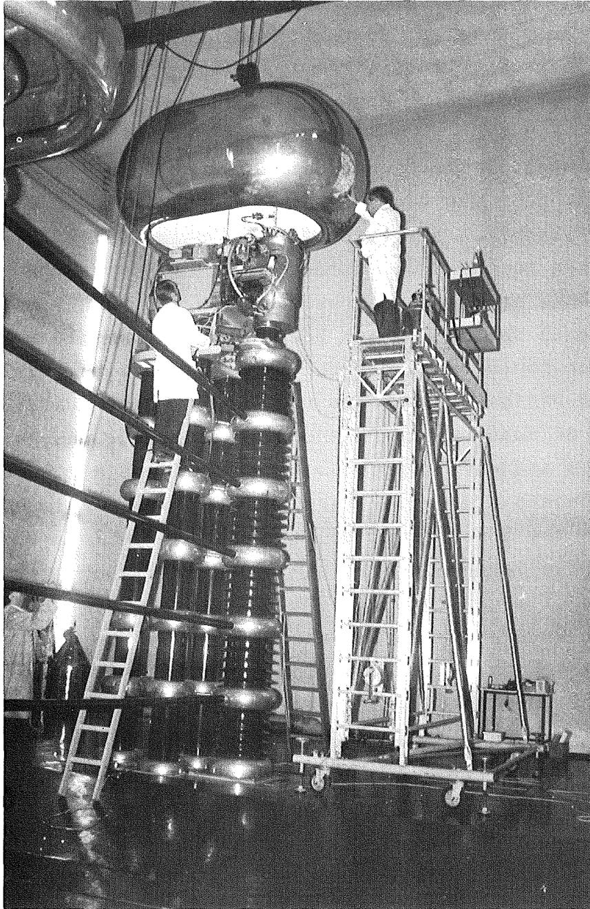
Fig. 5: Experimental set-up for the neutralization experiments at Grafschaft. Underneath the raised high voltage dome of the accelerator the cylindrical cryostat of the cluster ion beam source can be recognized.
