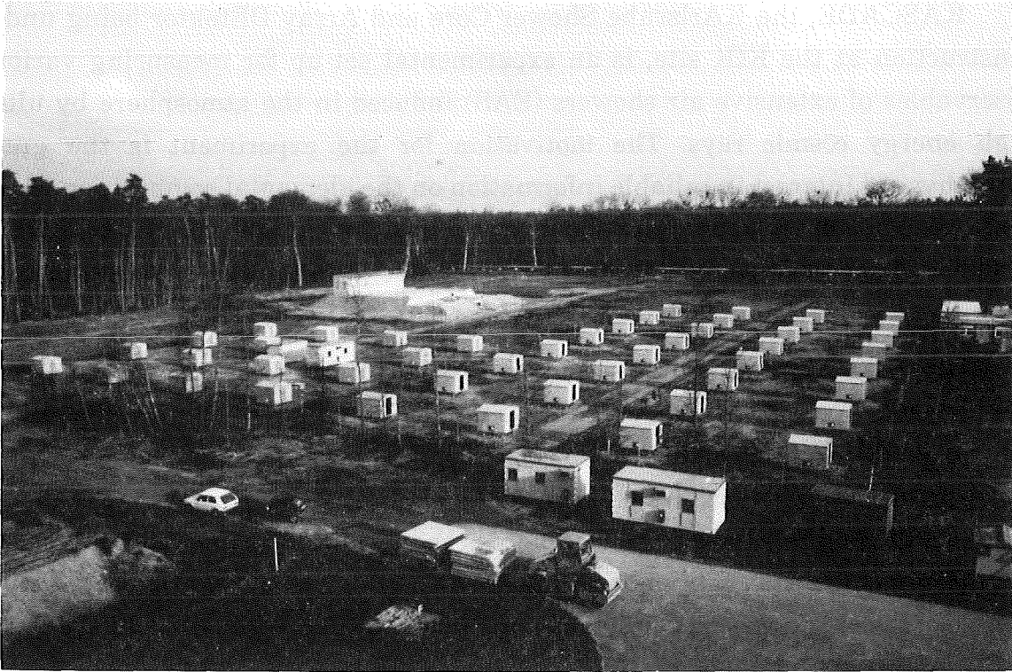
Fig. 1: View of the KASCADE-site by end of 1991. The picture shows three clusters of array detector stations in the foreground and the basement for the central detector and central electronic stations in the background.
