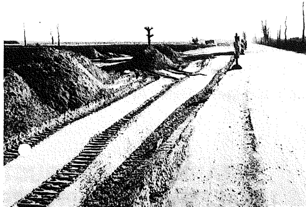
Preparing the SNR 300 construction site in Kalkar (1973).
