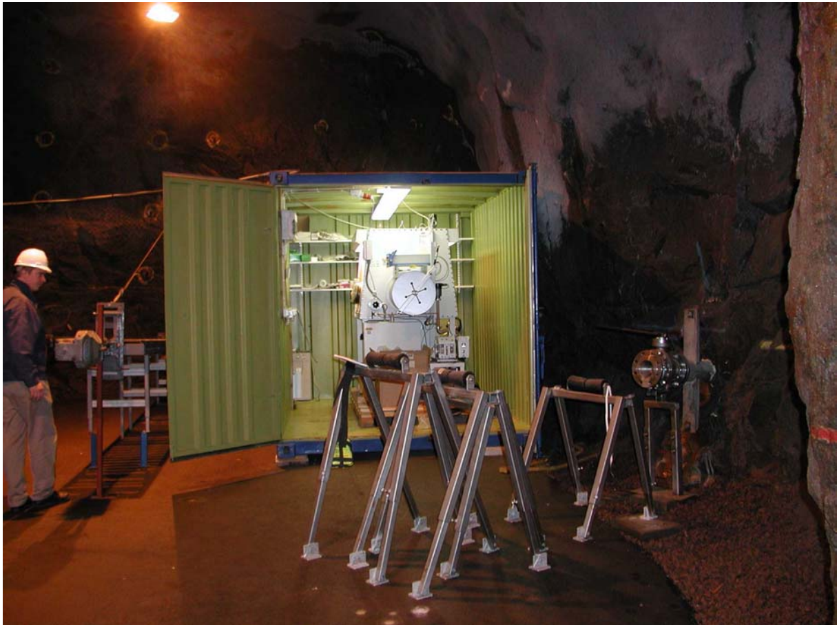
Fig. 3 INE glovebox installed in a container close to the CHEMLAB II drillhole The image shows the large main antechamber and the control unit and on the right side the CHEMLAB II drill hole lock
