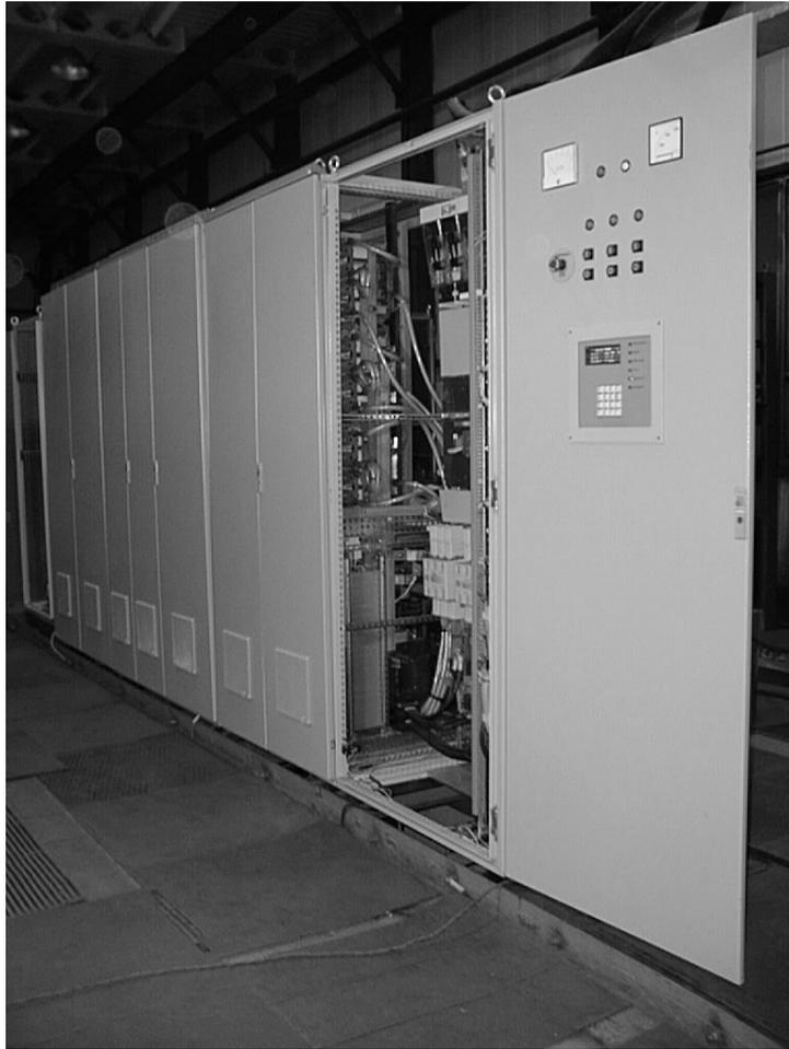
Fig. 6 View of completed cabinets of the SMES Modulator
