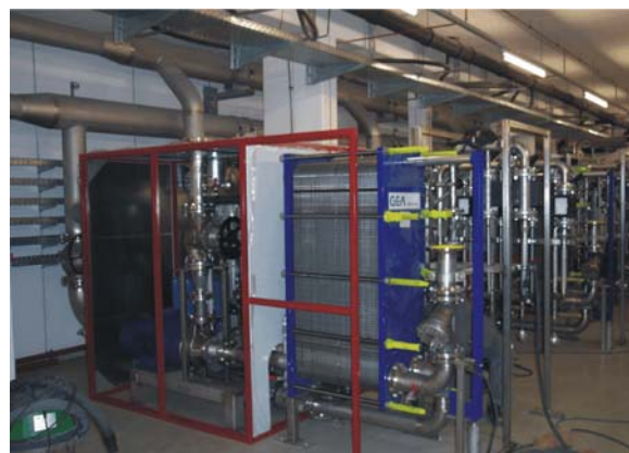
Fig. 6: Gyrotron cooling water modul [11].
