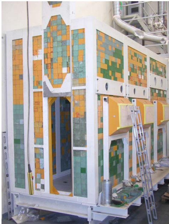
Fig. 2: New Materials Testing Cell under Construction.
