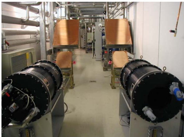
Fig. 4: View of the beam duct with MBWG mirrors and RF loads.
