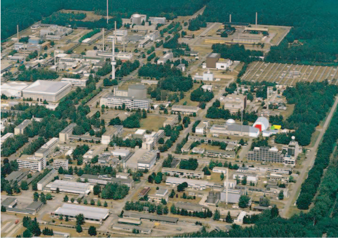
Figure 16: Aerial view of the site of Forschungszentrum Karlsruhe. A sketch of the location of the planned KATRIN experimental halls adjacent to Tritium Laboratory Karlsruhe (TLK) is superimposed.
