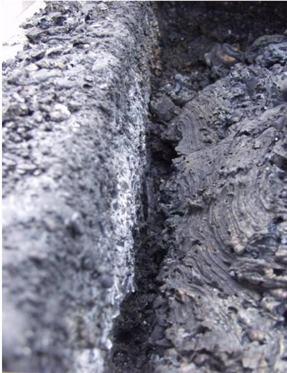
**Figure 3-22:** Gap at the concrete sidewall in area 8 (see Figure 3-18)
