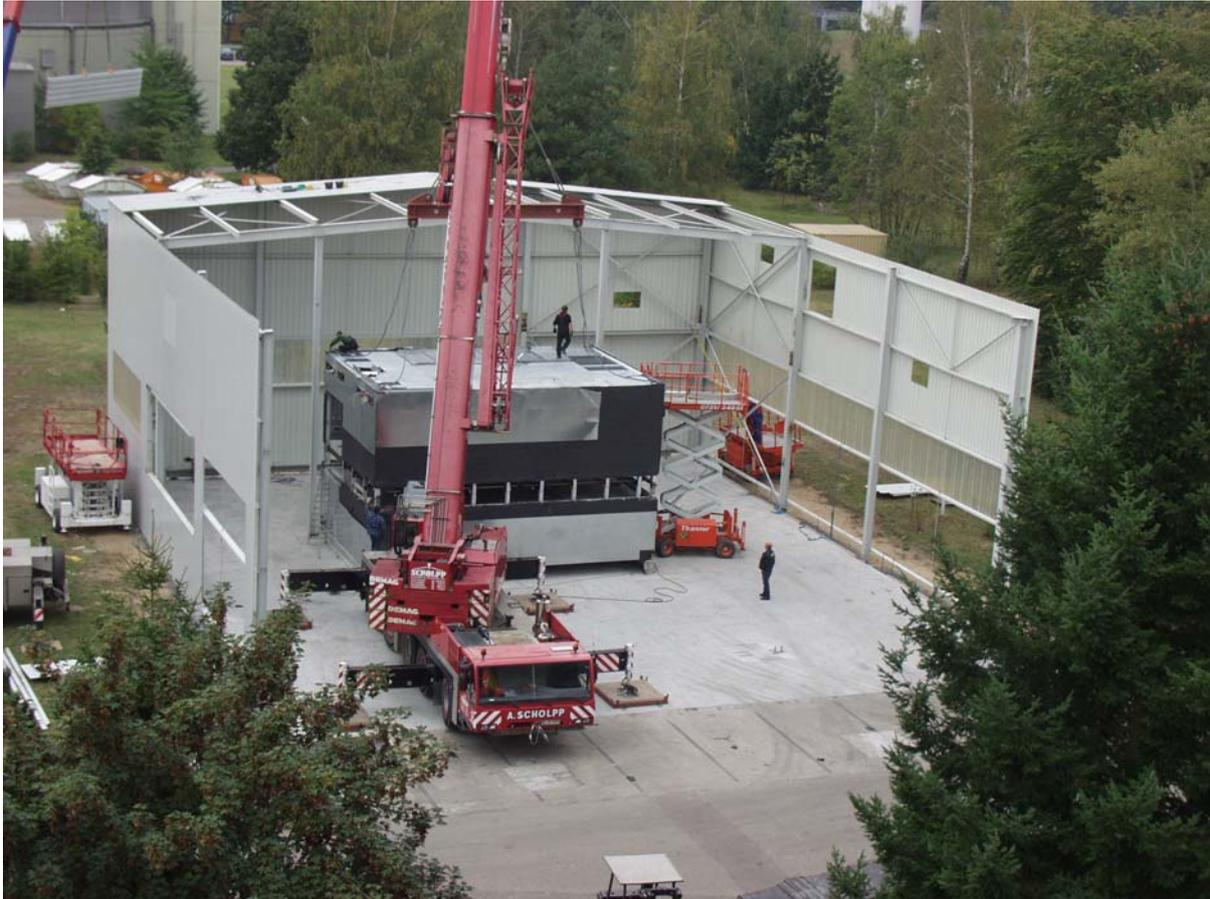
**Fig. 1b: Test cell Installation within the Experimental Facility**
