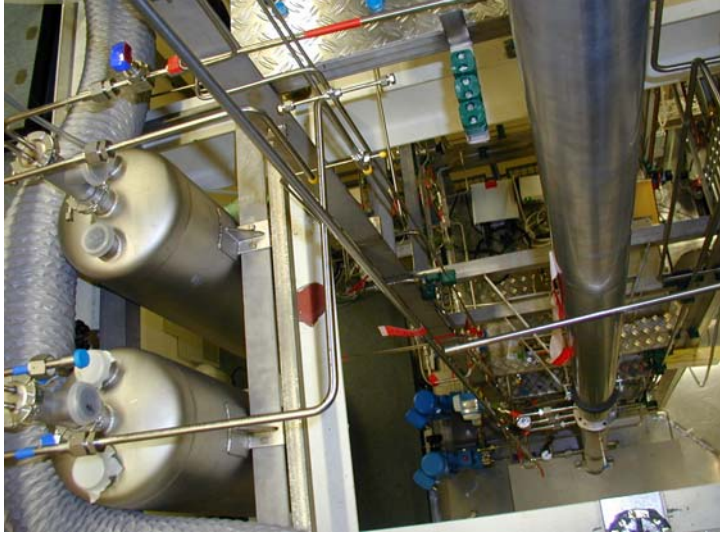
Fig. 2: The LPCE column of TRENTA facility.
