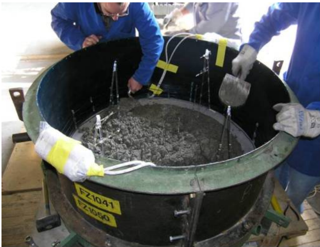
Figure 8: Fabricating the concrete crucible
