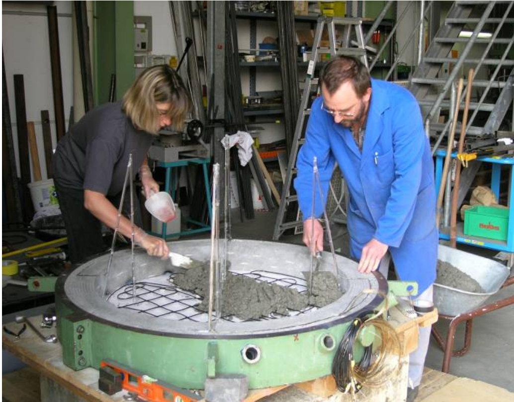
Figure 7: Fabricating the bottom of the concrete crucible
