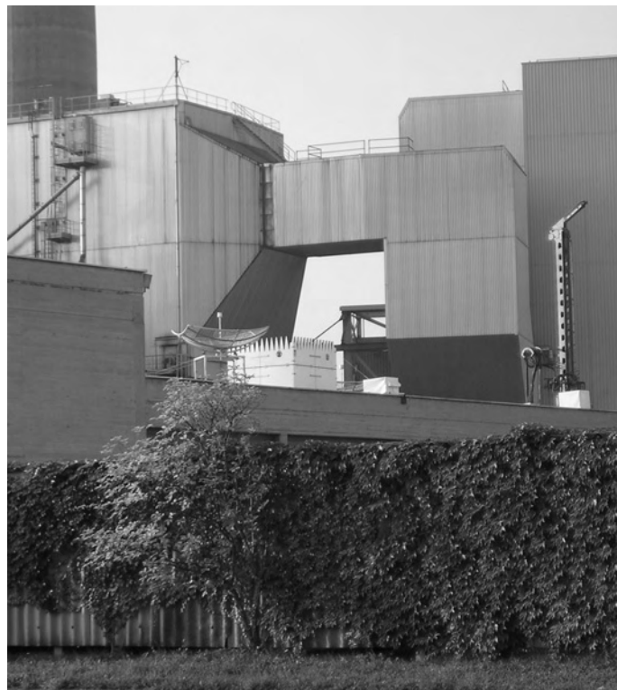
Figure 1. SODAR DSDPA.90-64 with RASS extension (Metek) at an industrial site in Linz on a flat roof 5 m above ground.
