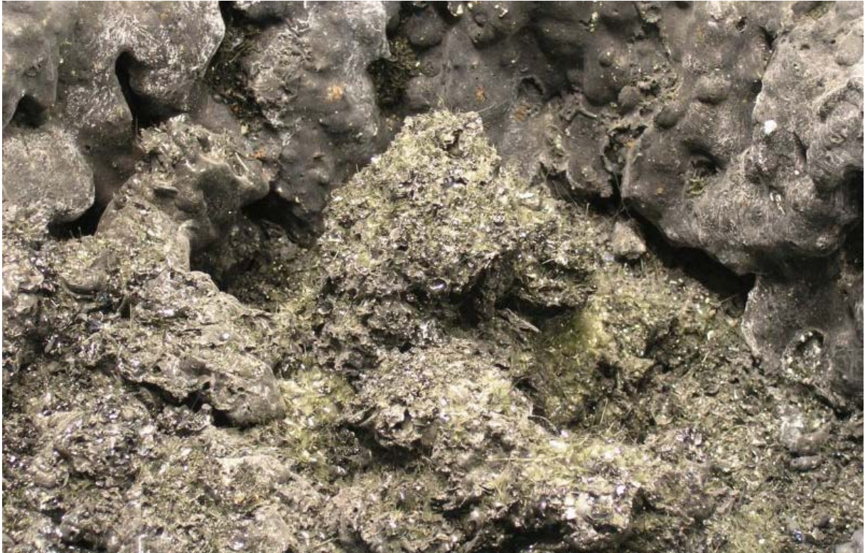
Figure 46: Close-up view showing the rough surface partly covered by ejected debris
