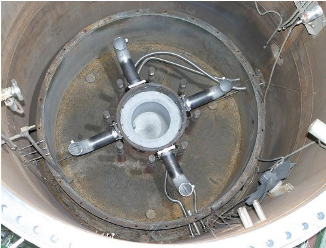
Fig. 12. View into containment vessel and cavity during assembly, G01-G06
