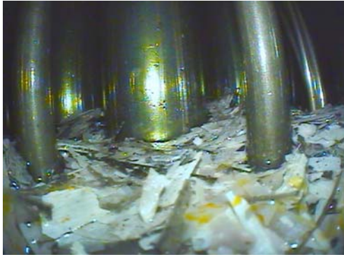
debris on bottom of separator
