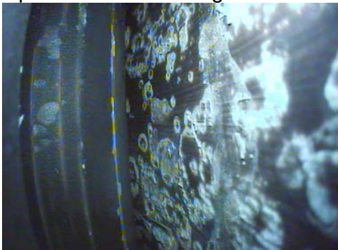
spallations at shroud at 850 mm
