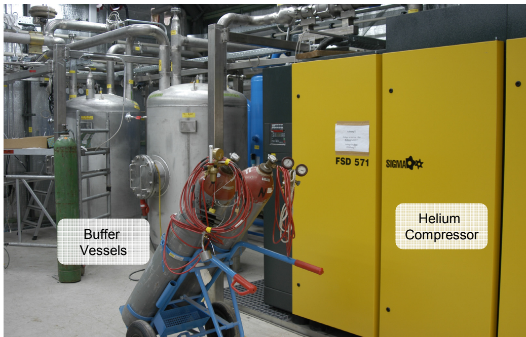
Fig. 2: Installation in new auxiliary hall (building 508).
