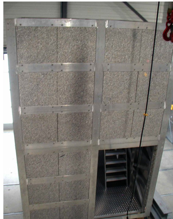
Fig. 2: „ECRH tower“ for shielding and installation of the mirrors near to W7-X.
