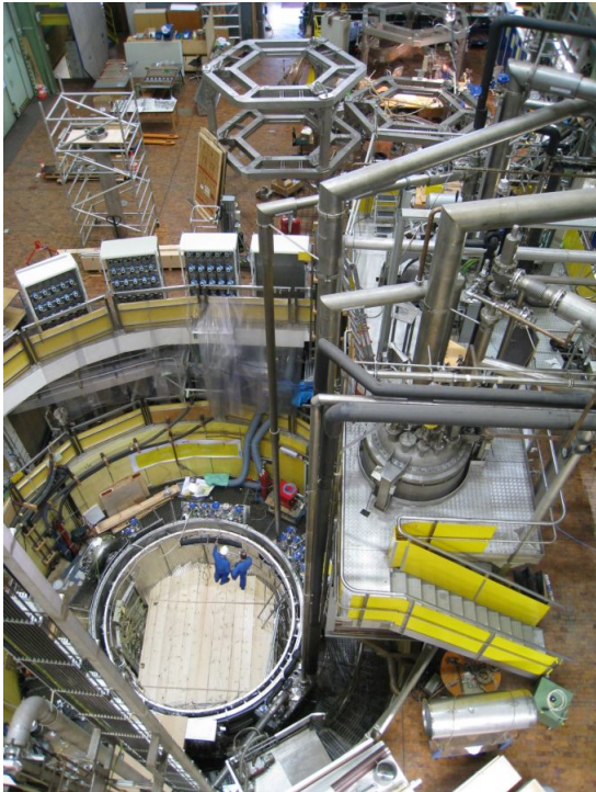
Overview of TOSKA facility during preparation for W7-X coil testing
