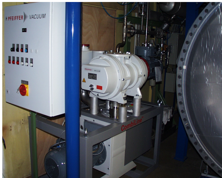
Fig. 1: The new regeneration vacuum pump station of TIMO-2.
