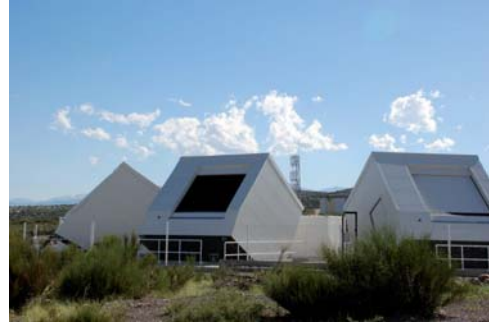
Fig. 2. Photo of the 3 HEAT telescopes tilted upward, end of January 2009. In the background the telecommunication tower of Coihueco is visible.
