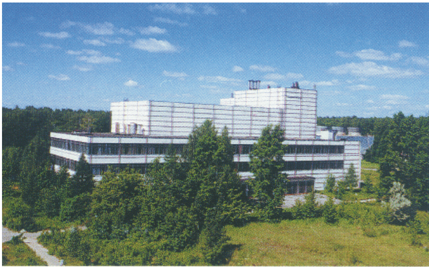
Fig. 2-1 Reactor building of BOR 60.
